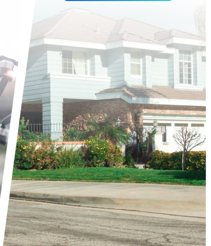
Home Backup Power
